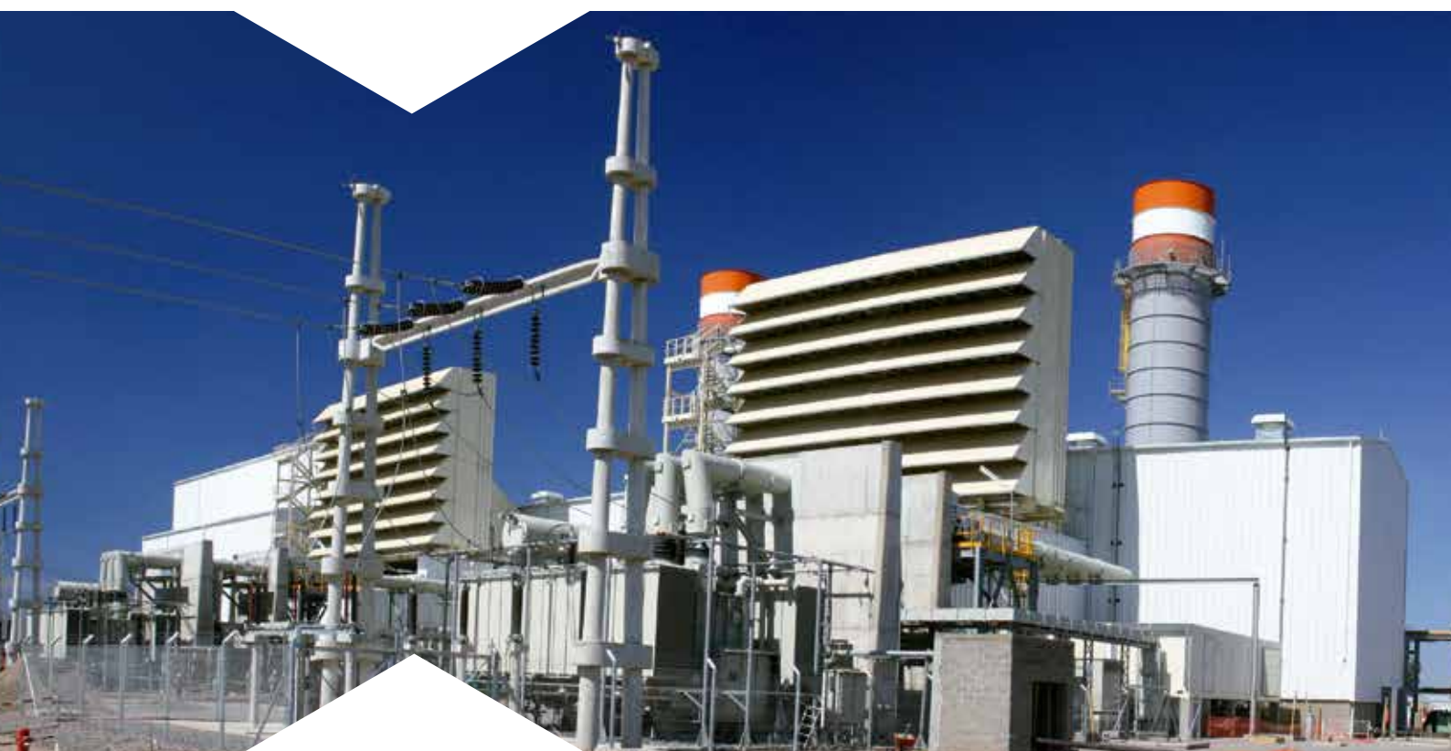
Combined Cycle Power Plant (Pilar-Córdoba) 460 MW
